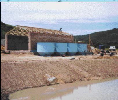
Packaging Plant Buiding (Dwese WSS)
