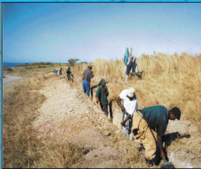
Trench excavation - July 2001 (Dwese WSS)
