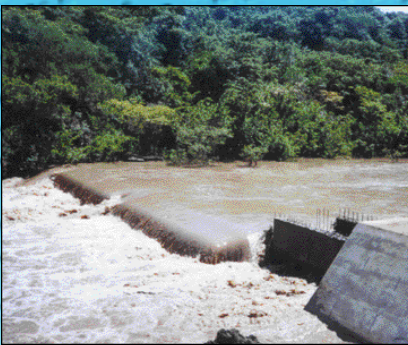
Weir wall - Nov 2001 (Dwese WSS)
