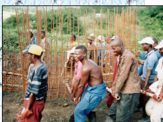
Prefixed reinforcing for intake tower Umzimvubu Project
